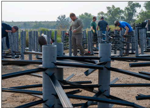
Club members helped to assemble the fish habitat structures.
